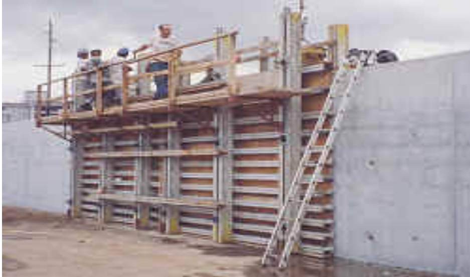
Wall Forms are Used to Place Concrete for vertical walls.
